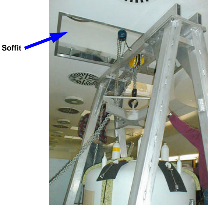
Figure 4.2. A Soffit (including gantry used for installation)
