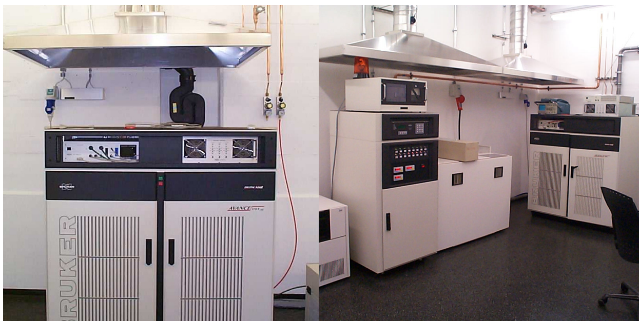
Figure 6.3. Commercial Ventilation Systems
