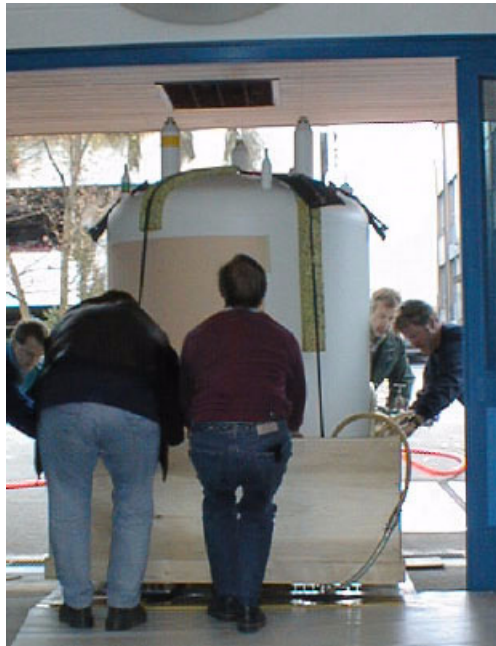
Figure 3.1. Moving the Magnet on Air Skates Through the Laboratory Door
