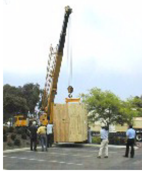
Unloading the magnet crate off the truck and positioning it on the ground for uncrating.
