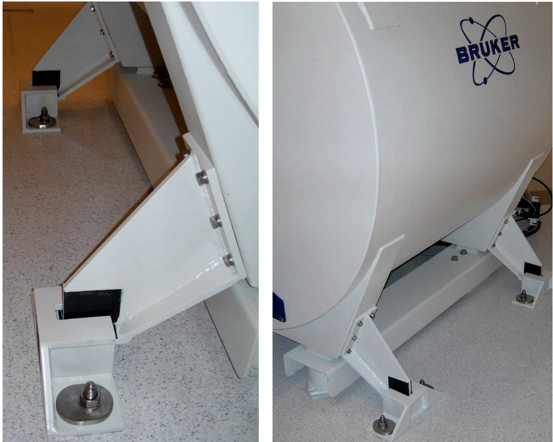
Figure 6.13: Seismic protection system at the magnet.
