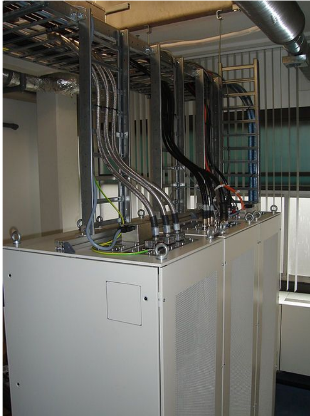
Figure 6.19: Construction of cable carrying system
