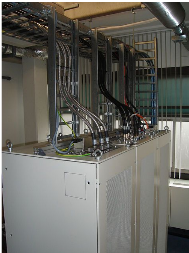
Figure 6.19: Construction of cable carrying system
