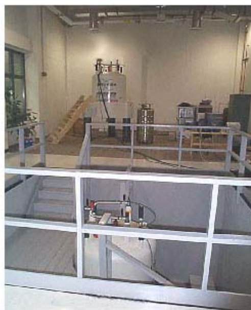
Figure 8.5. Example of a Magnet Pit
